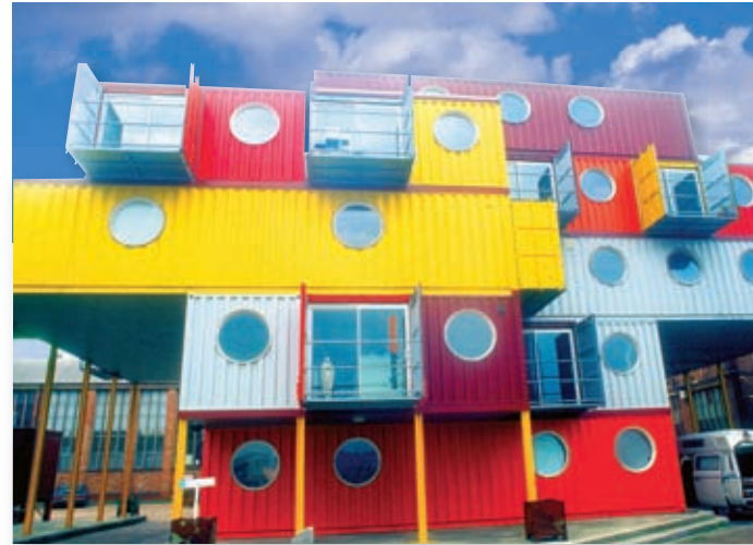
Container City, in East London, UK, is a development of buildings made from recycled shipping containers.
